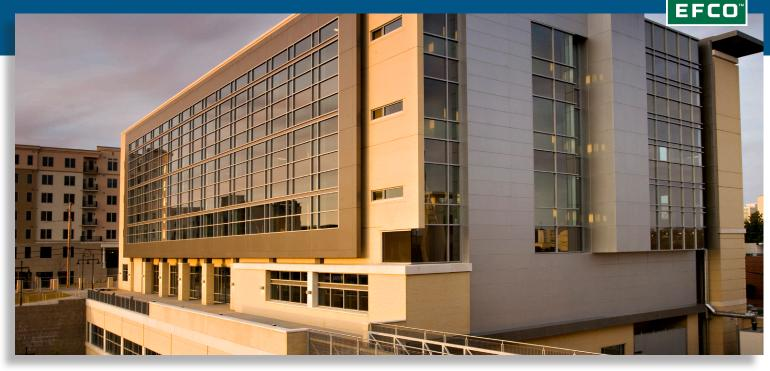
Outside Glazed - Captured • 2-sided SSG, and 4-sided SSG The 5600PG is a versatile curtain wall system that can be provided in stock lengths, Pre-glaze capability for customers, and Factory fabricated/assembled & glazed. Options available for enhanced performance and fewer installation steps.
